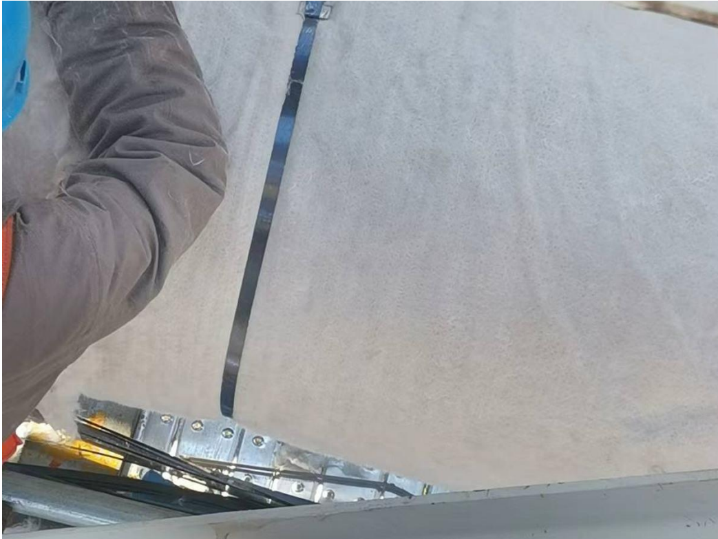
BASF-YPC · Medium-pressure steam line
